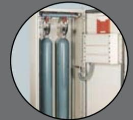
3. The clean agent extinguishing system's nitrogen gas cylinders are pressurized so that the weight and space requirements are minimized
